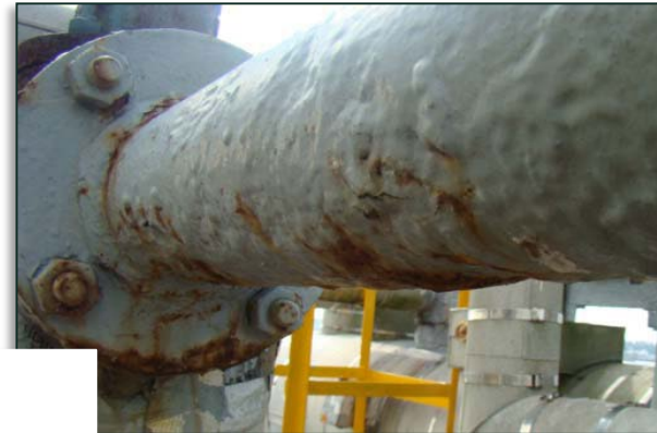
Incorrect application of a coating system on a carbon steel \text{NH}_3 pipeline in urea plant
