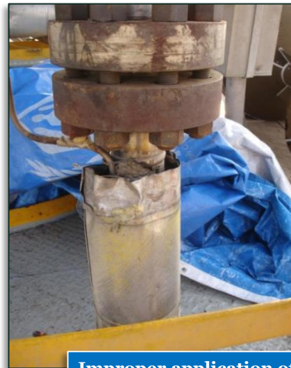
Improper application of insulation sheeting
