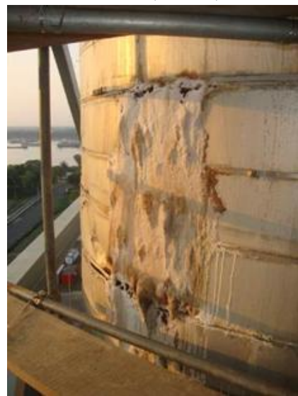
Figure 1: Crystallized product visible on cover sheeting insulation urea reactor
