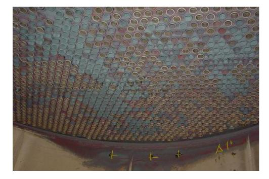
Photo 8: Bottom tubesheet after 860 days on stream shows a bad liquid distribution
