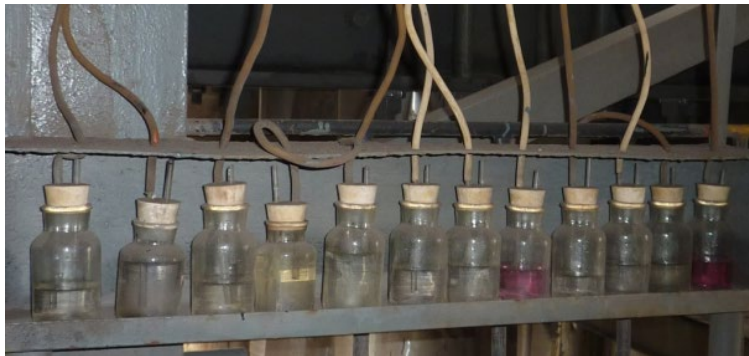
Figure 8: A typical passive leak detection system
